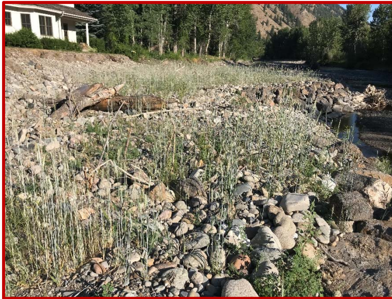
Figure 20. Photograph depicting an example of a constructed floodplain bench with vegetation plantings and a rock toe
