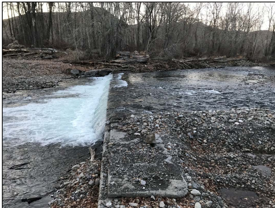
Figure 8. Photograph depicting channel-spanning concrete sill at District 45 diversion, November of 2018.
