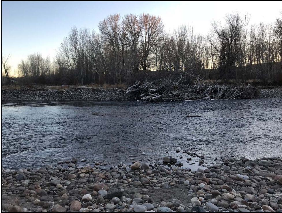
Figure 12. Photograph depicting debris jam and gravel deposits that filled in excavated side channel on the west side of the river, in November 2018.
