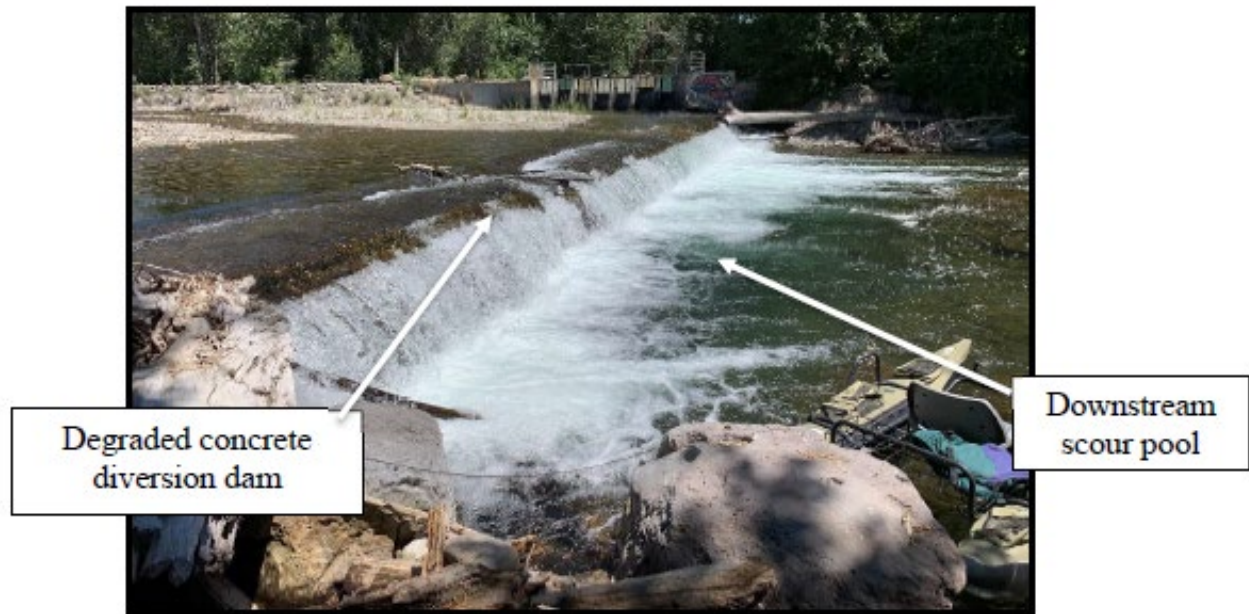
Figure 1. Existing condition of Diversion 45 on the Big Wood River, Bellevue, Idaho.
