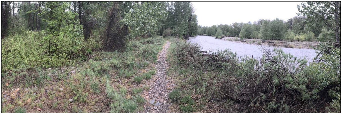
Figure 9. Photograph depicting constructed berm that limits floodplain inundation and flood water dispersal in the Howard Preserve.
