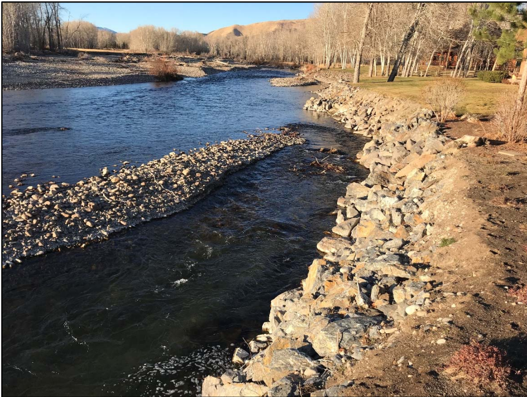
Figure 17. Photograph depicting transverse depositional bar promoting high near bank shear stress, and rock rip rap treatment installed in response to severe land loss and bank erosion in 2017, Riverside Subdivision.
