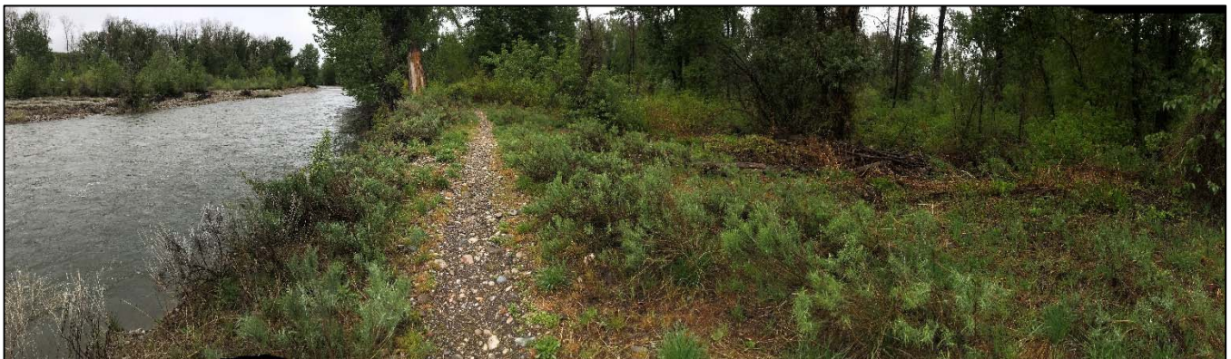
Figure 10. Photograph depicting constructed berm that limits floodplain inundation and flood water dispersal in the Howard Preserve.
