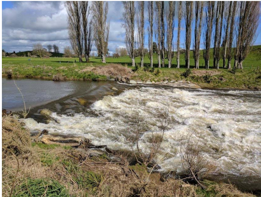
Figure 19. Example photograph depicting a rock ramp boulder structure (Source: Paul Franklin).
